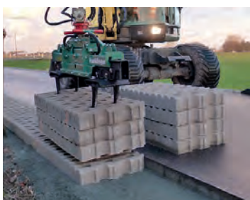
Installing first layer and picking up remaining three layers
