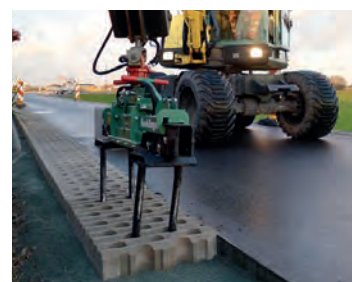
Working effectively Up to four times the laying output
