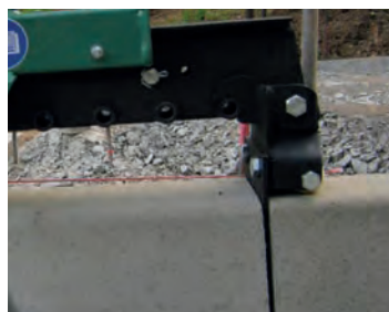
Precise kerb laying Special gripping jaw allows exact positioning of kerb
