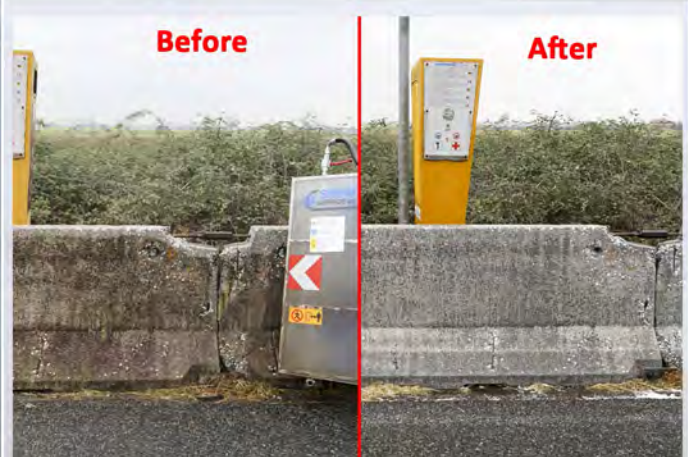
EFFECT TO THE ROTARY NOZZLES ON THE WALL
